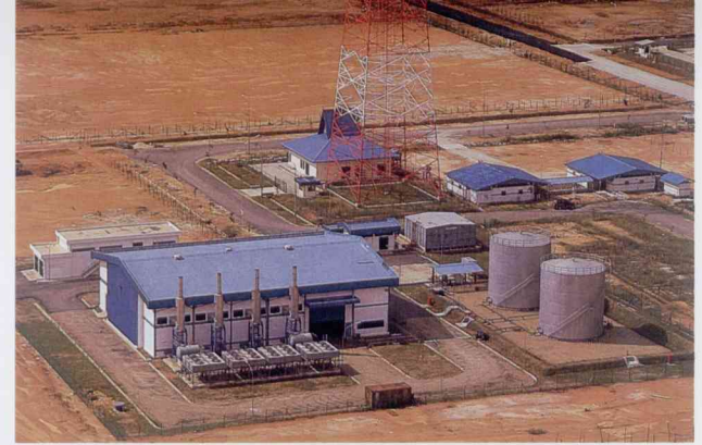
An aerial view of utilities, factories and dormitories in the Bintan Industrial Estate.
