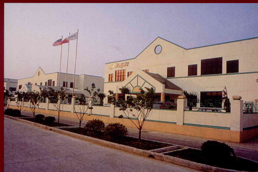
Seagate Technologies' Wuxi Plant.
