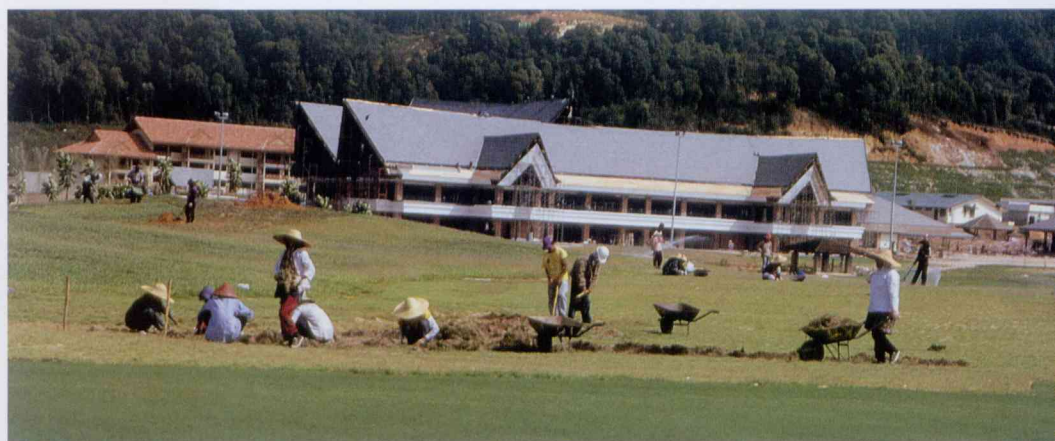
Workers preparing the golf course at Batamindo Executive Village.
